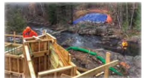
Snowmobile bridge construction.
